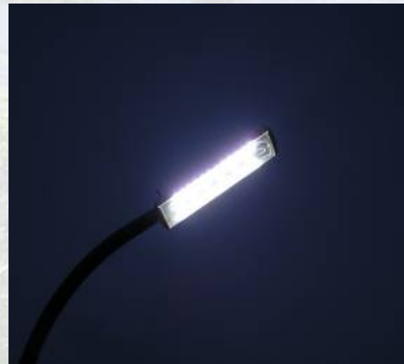
Street light replace from Mercury type(400W) to LED type(100W)
